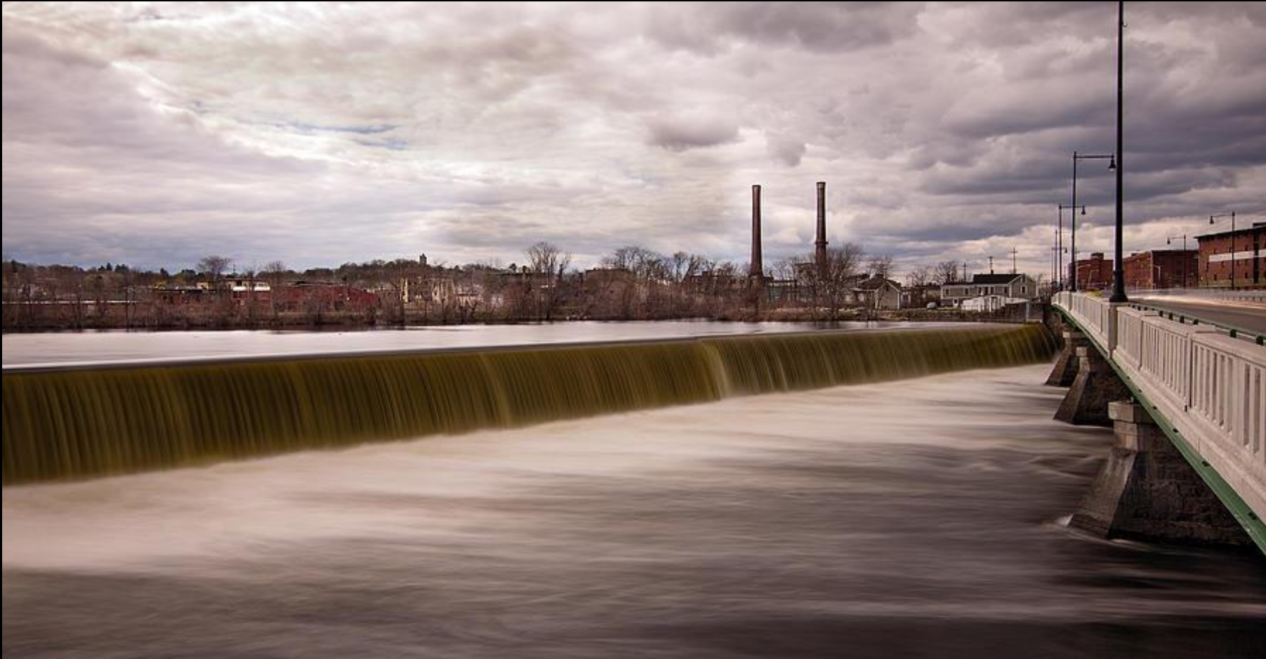
Great Stone Dam, Lawrence, MA. Erected 1815 by the Essex Company. The largest made-made structure of its time: 900-feet long, 30-feet tall, 35-feet thick
